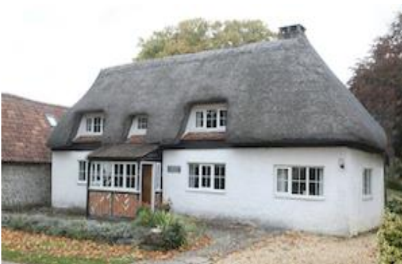
Figure 16: Conservation Area Building (2020).
